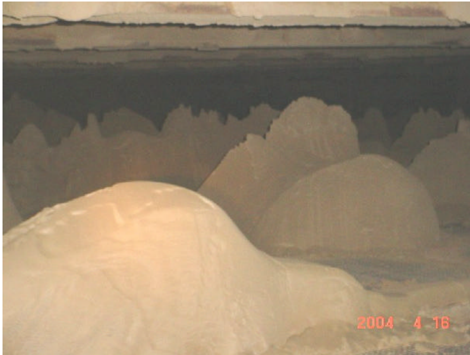
Figure 8b. Deposits of Ash on Turning Vanes
