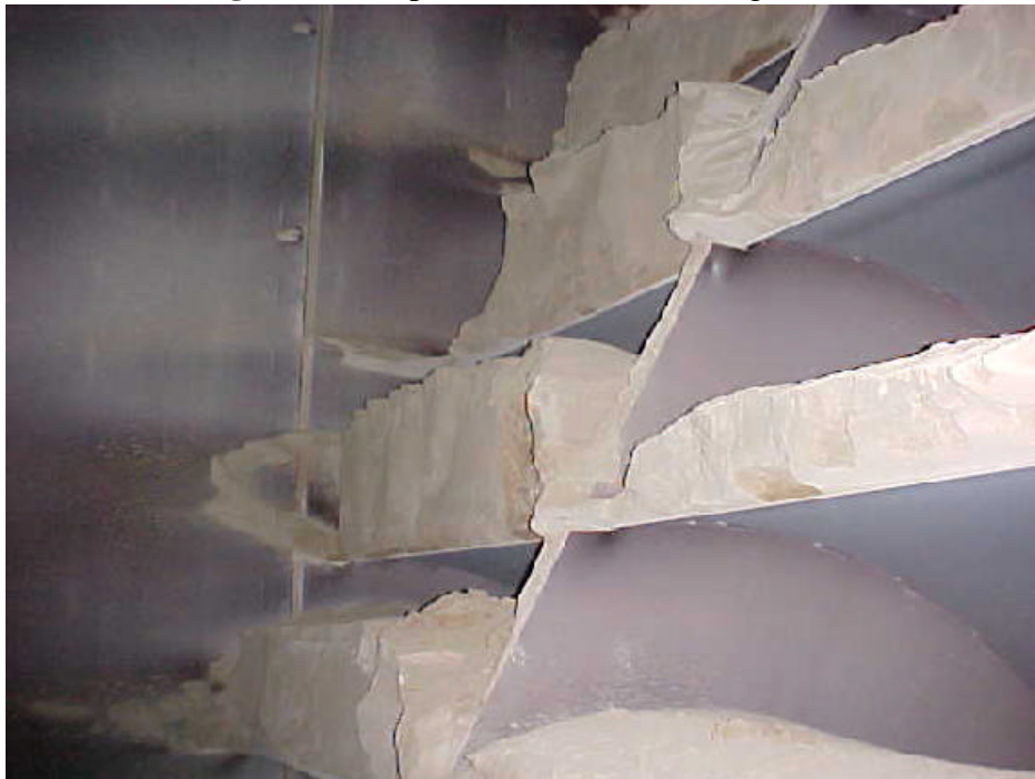
Figure 8b. Deposits of Ash on Turning Vanes
